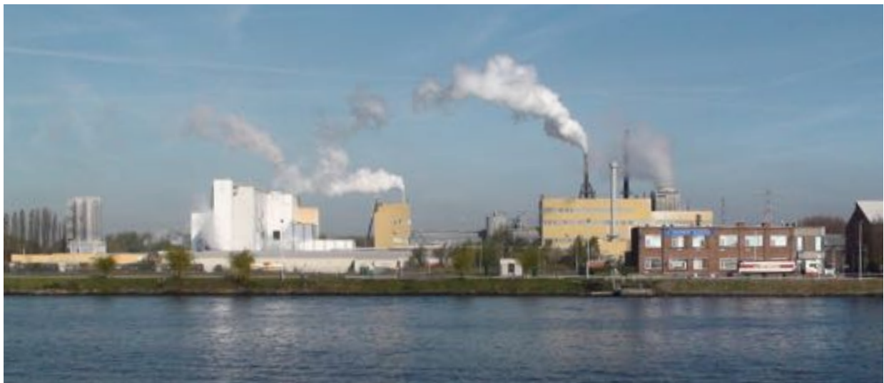
One of the six production units operated by Kronos International, Inc. with headquarters in Dallas and main office in Leverkusen, is located in Langerbrugge in Ghent, Belgium.
